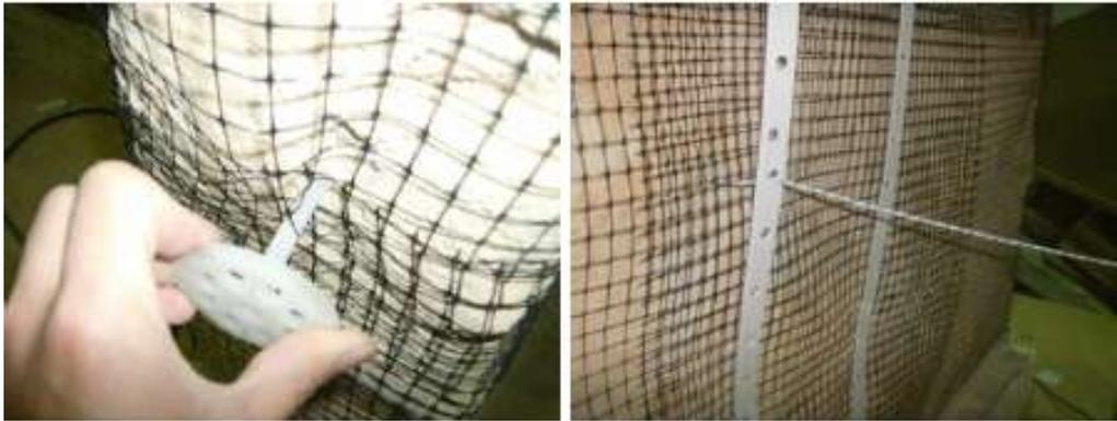
Figure 3-5 Reinforcing masonry/adobe walls with geo-mesh (Source: world housing tutorial)
