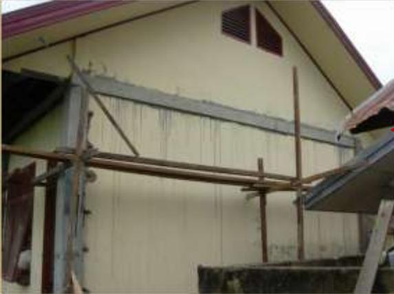
Gable walls are not recommended in earthquake prone areas. They should be removed and replaced with other materials such as CGI sheet. In case gable walls are unavoidable, Gable beam properly connected with the columns shall be placed.
