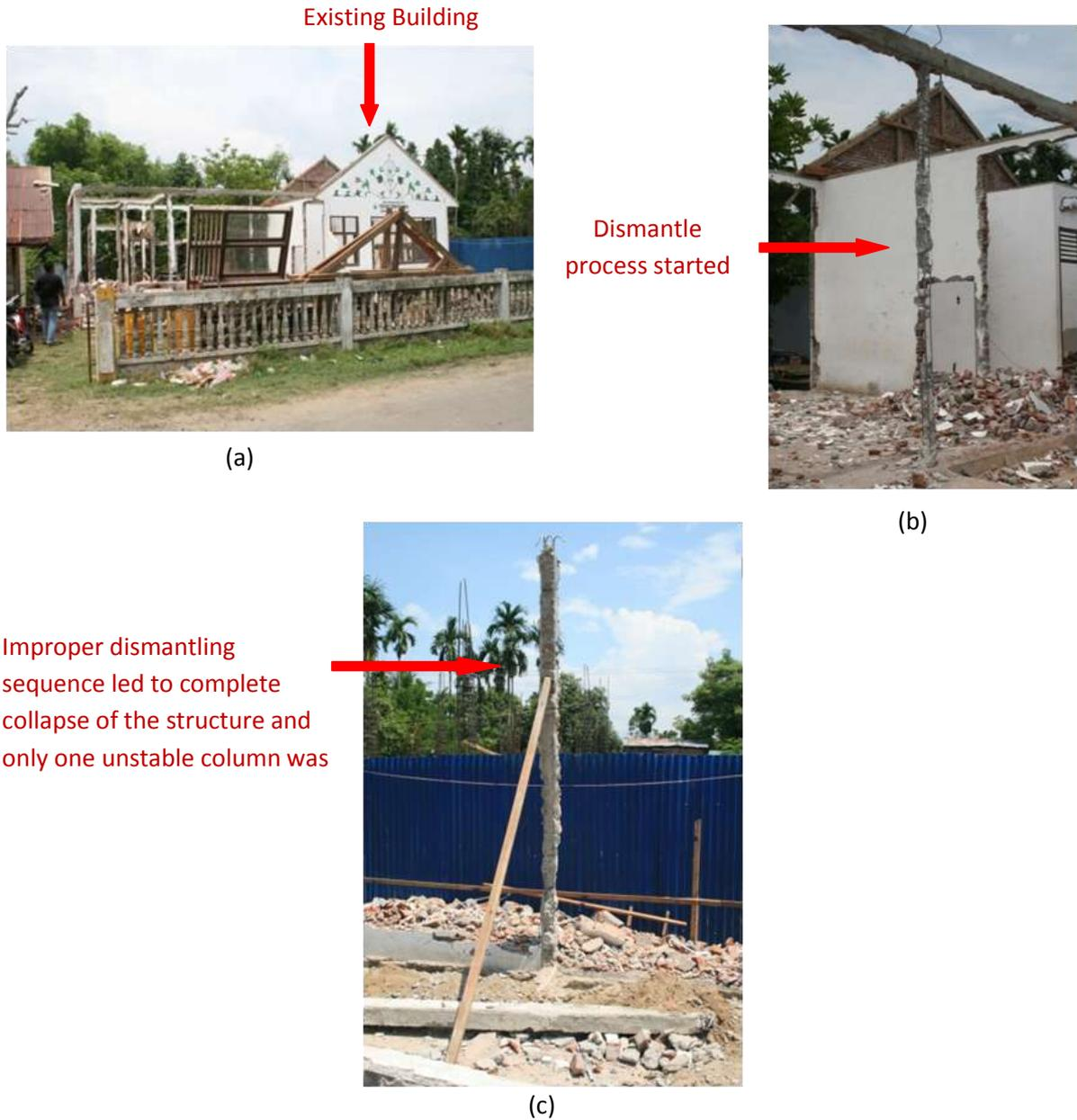
Figure 2-1 Improper construction sequence led to complete collapse of the structure during retrofitting
