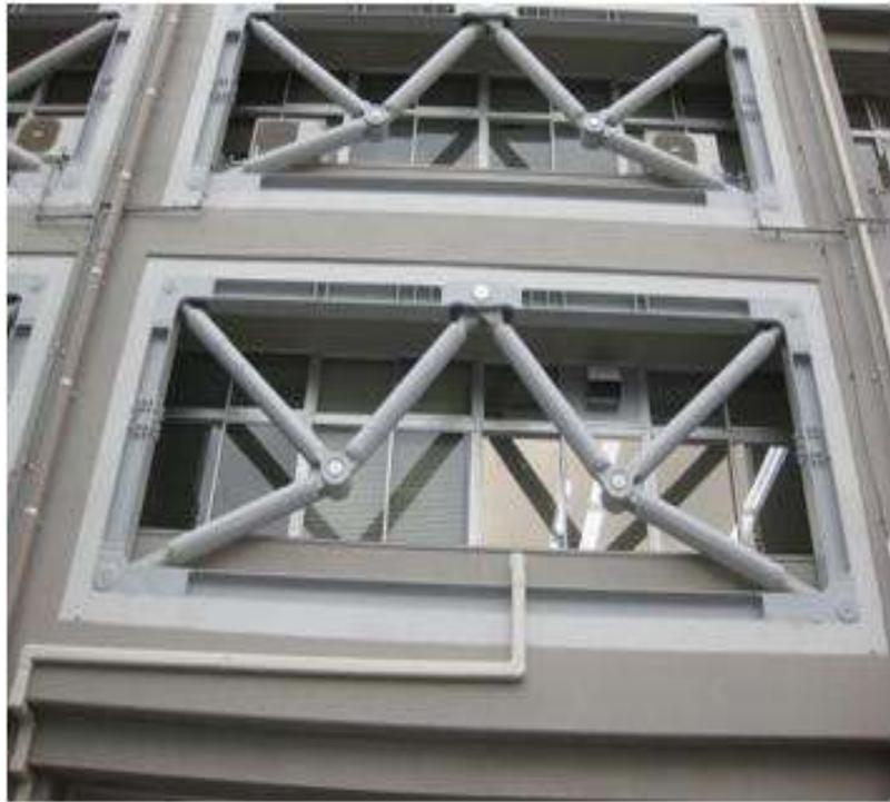
Figure 3-4 Introduction of dampers in existing RCC structure
