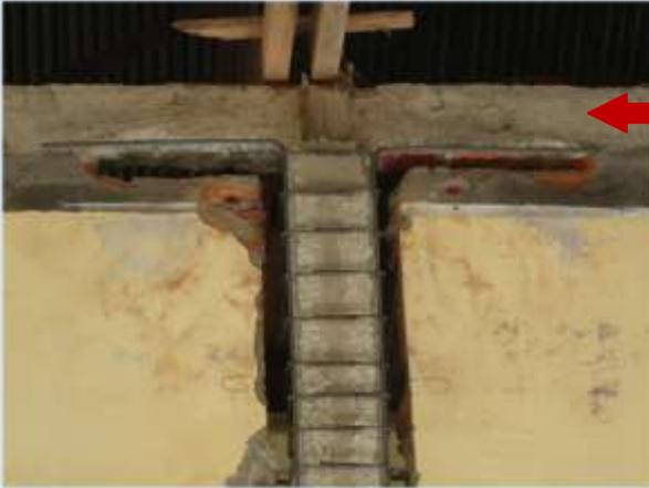
Beams need to properly connected with the columns and the reinforcement of column should continue toward the beam.
